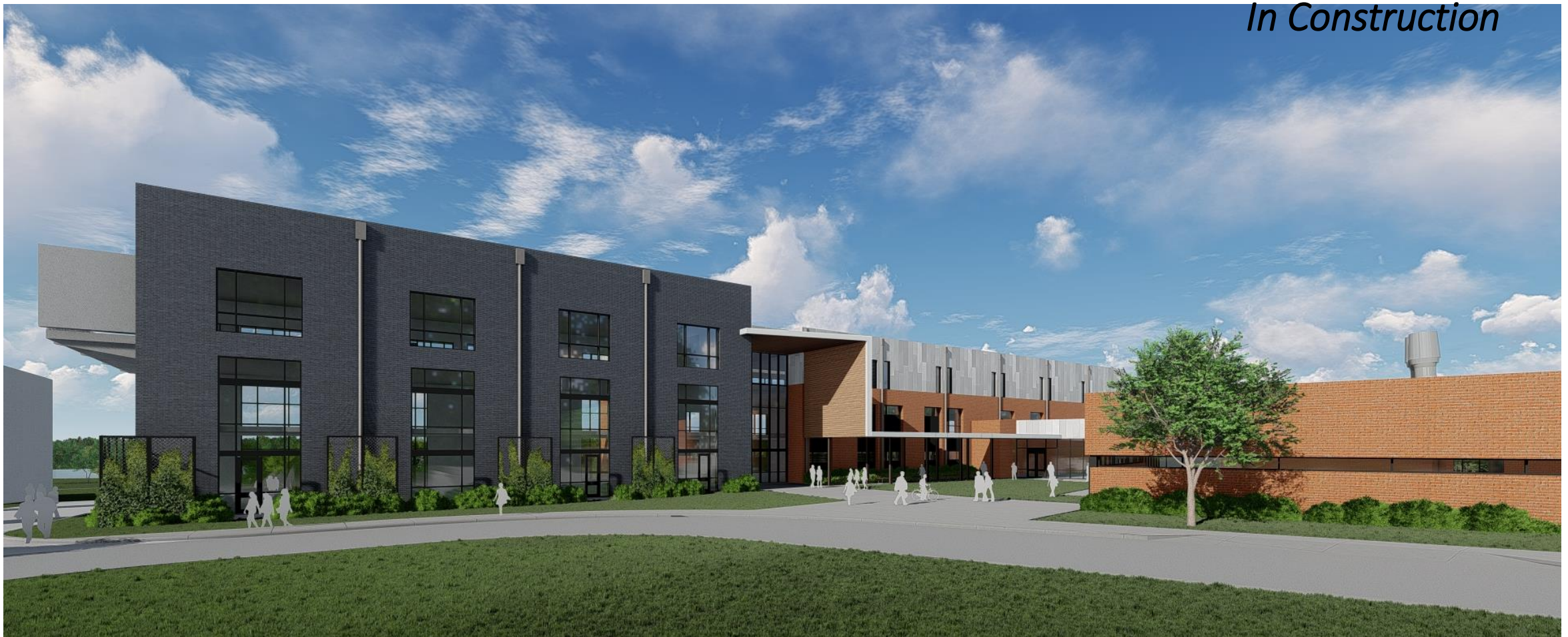
North Elevation and Courtyard
