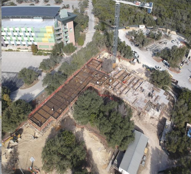
2nd Floor Slab Formwork
