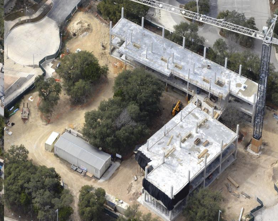
3rd Floor (Final Floor) 3 Story Concrete Structure Complete
